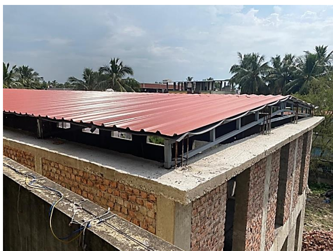
Dec 14 th – roof sheets fixed
